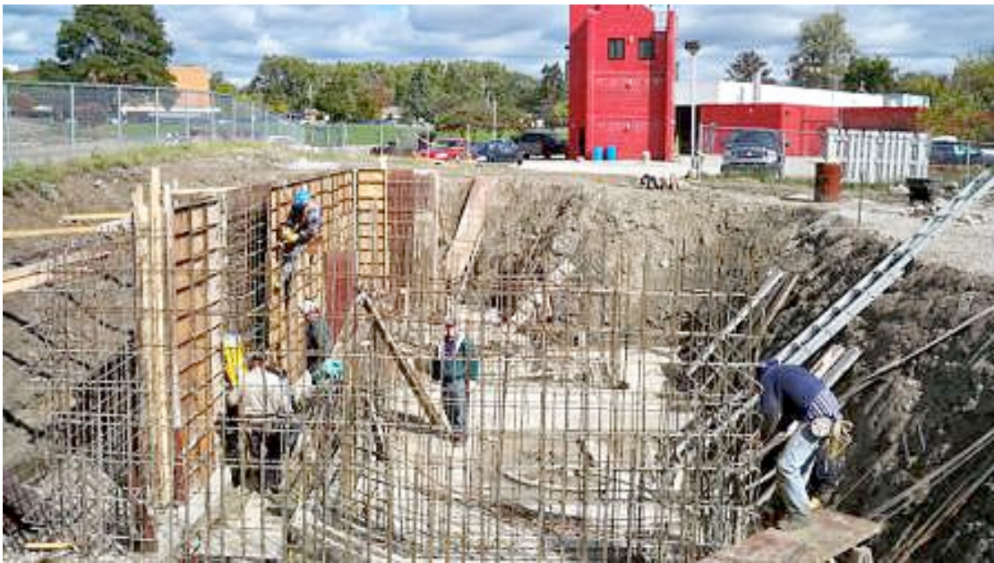
The Southfield trench rescue simulator under construction.
